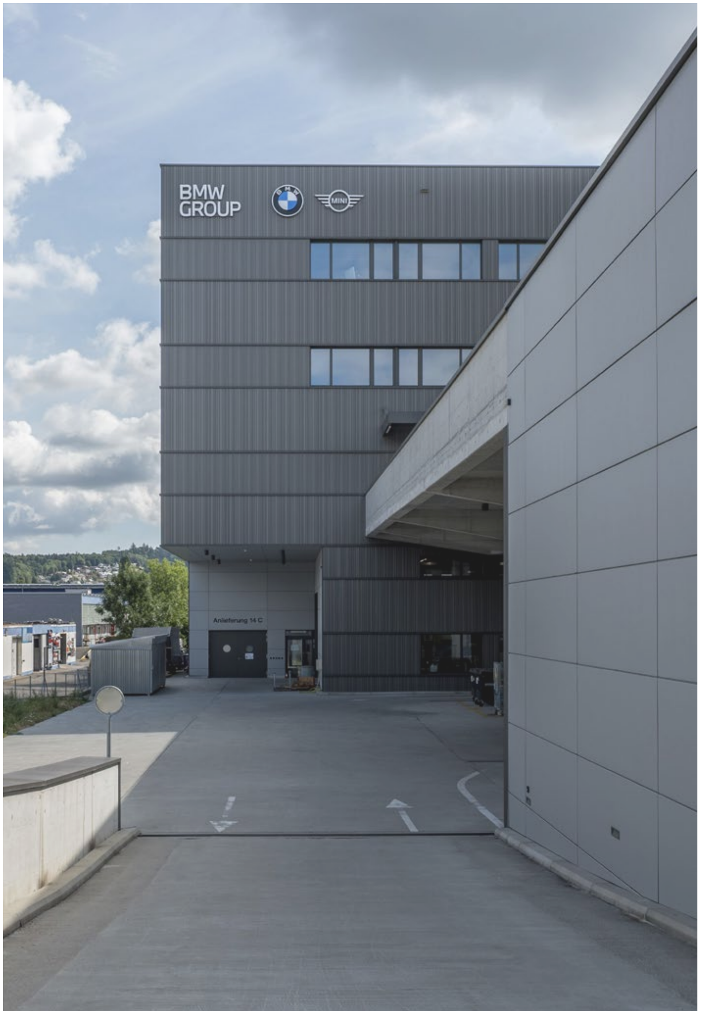
Photo: Brühlmatten 14a, b, c, Zofingen (AG)
