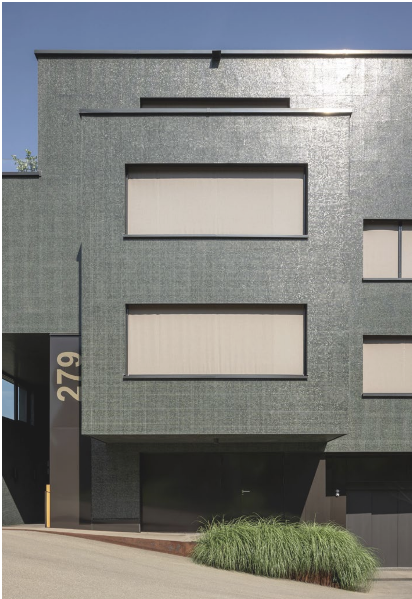
Photo: Forchstrasse 275, 277, 279, Zürich
